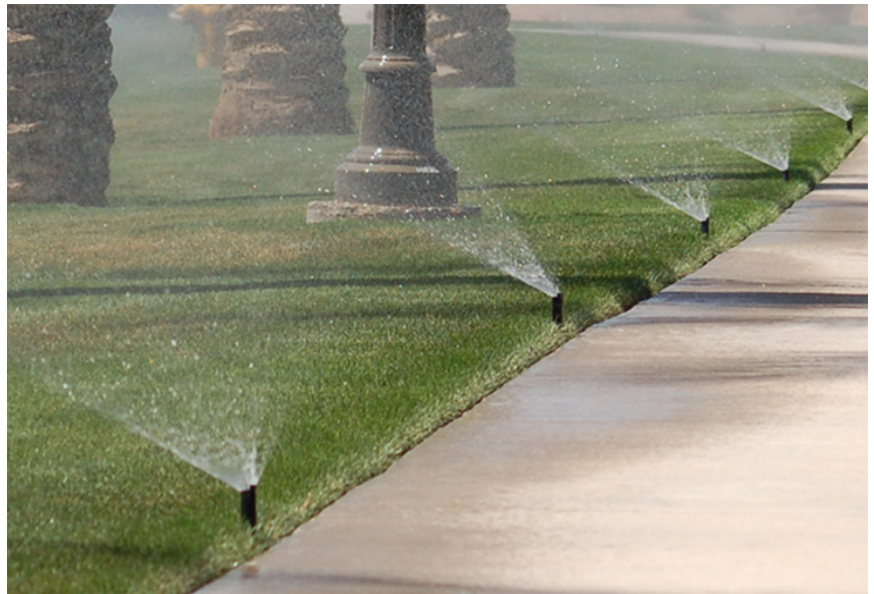
Make sure all nozzles are pointing in the right direction to ensure the intended area is being sprayed
