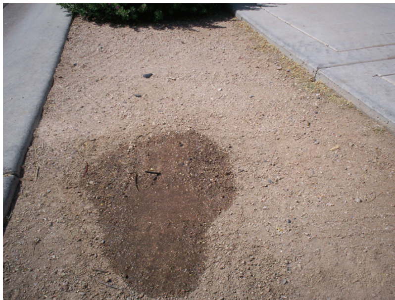
It is important to plug all unused emitters even though the water loss is insignificant compared to water used to irrigate turf areas.
