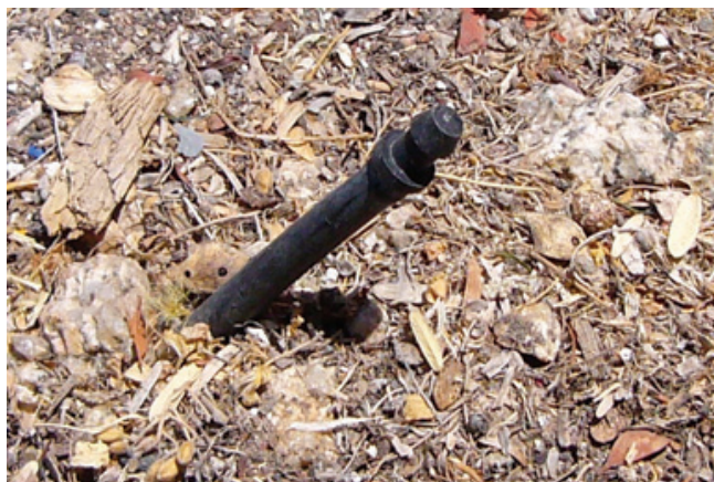
A drip tube that has been capped.
